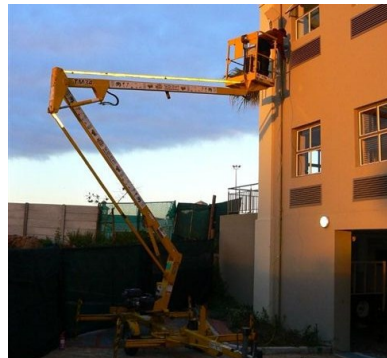
Installation in progress
