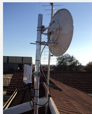
Installation at engineering office
