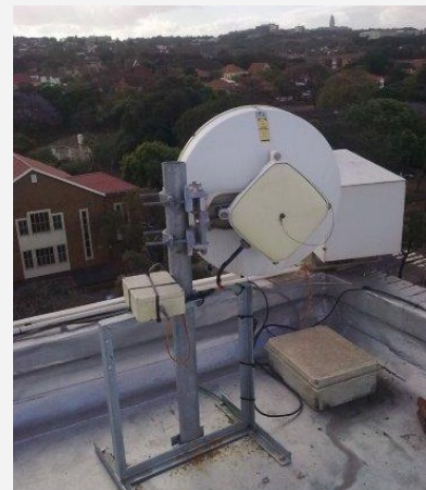
Gigabit wireless Bridge Point-to-Point high capacity network connectivity between, medical school and science block.
