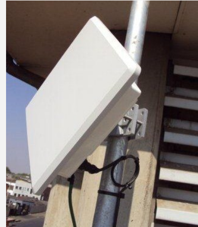
Proxim broadband wireless services last mile access, Point-to-Point or Point-to-MultiPoint solutions. These connect faculties in the 3 to 10 km radius of the main campuses.
